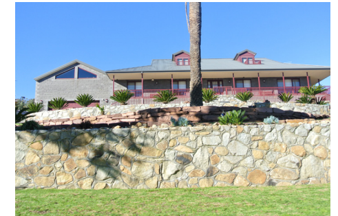
Example Four: Retaining Walls
