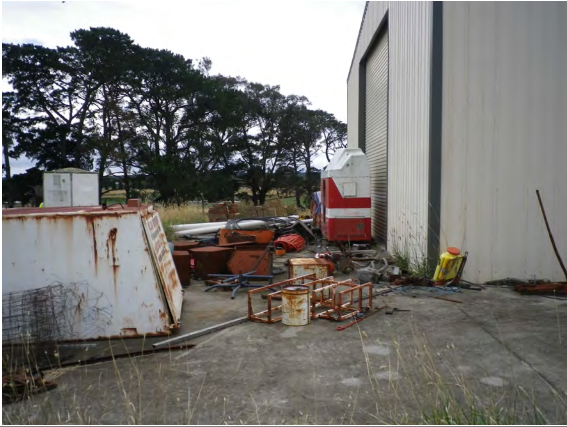
Plate 13 - Property 35, large shed for storage of machinery and heavy equipment. Oil containers located on hardstand area surrounding the shed.
