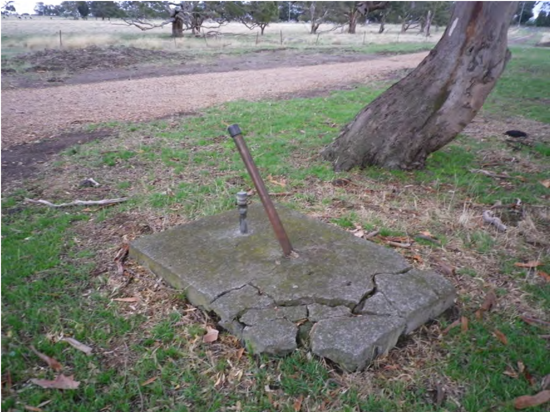
Plate 4 - Property 31 potential underground storage tank, with fill / observation points.
