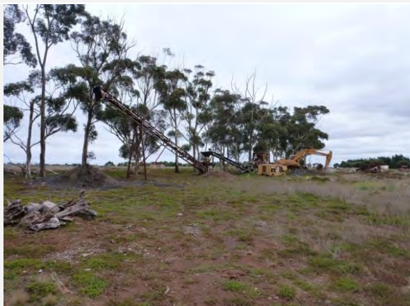
Property 35 Aggregate sorting equipment along southern boundary.
