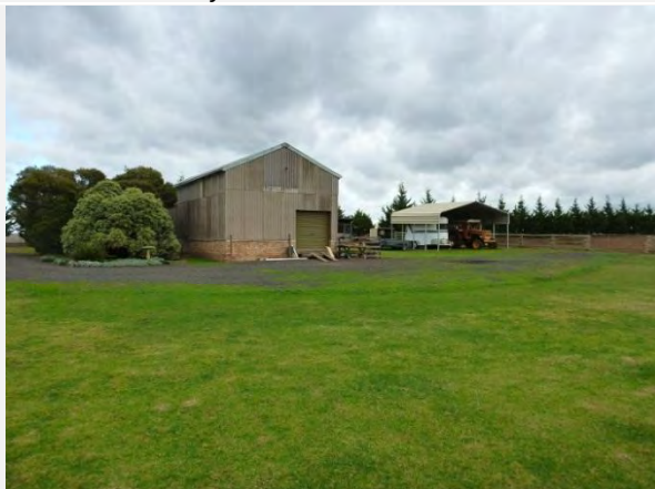
Property 4 Sheds containing suspected ACM sheeting.
