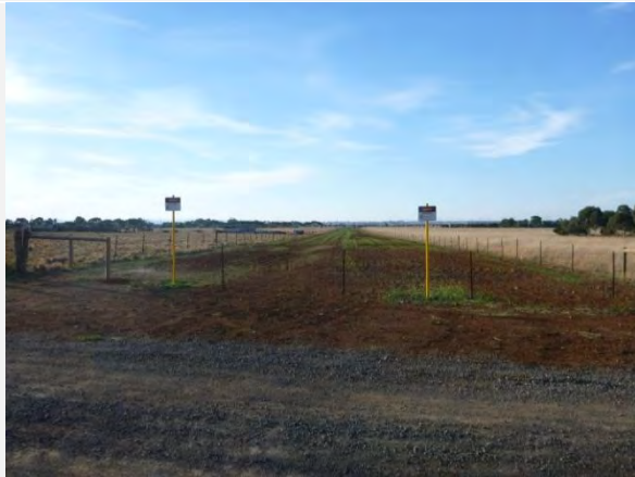
Property 84 Gas pipeline intersecting site.
