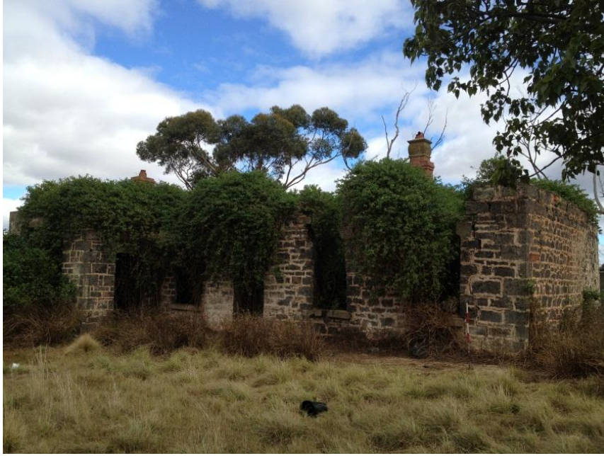
Plate 2: Doherty House (HO36) (photo faces south east).
