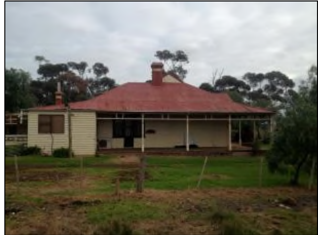
Plate 2: Study area facing south within Property 33, showing area of residential development.
