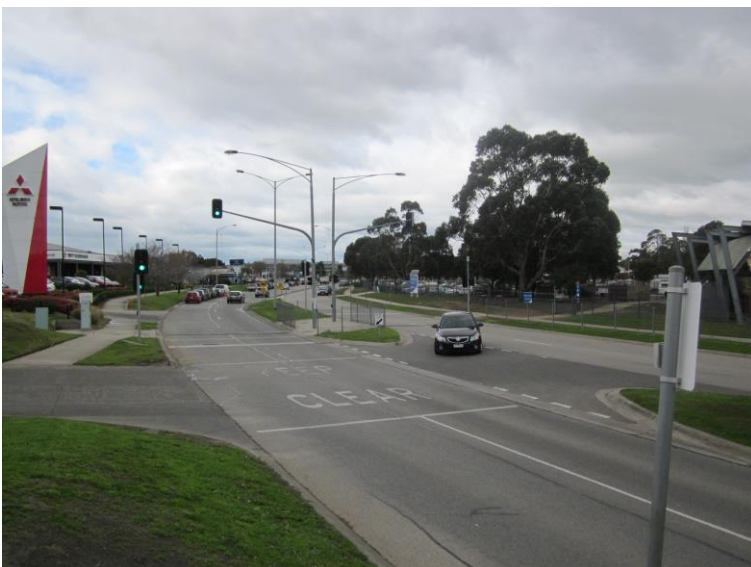
Figure 3-4 Kangan Drive (facing east)
