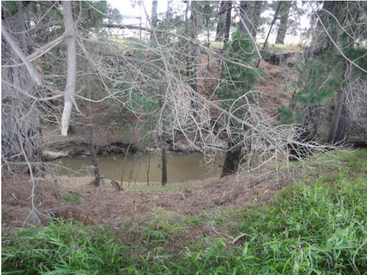
Figure 19 Section of Cardinia Creek (110 Smiths Lane), note the steep banks and vegetation dominated by Monterey Cypress pines.
