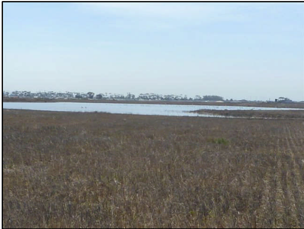
Plate 11: View of the dam outside the eastern boundary, forming a catchment for the central drainage line, facing east.
